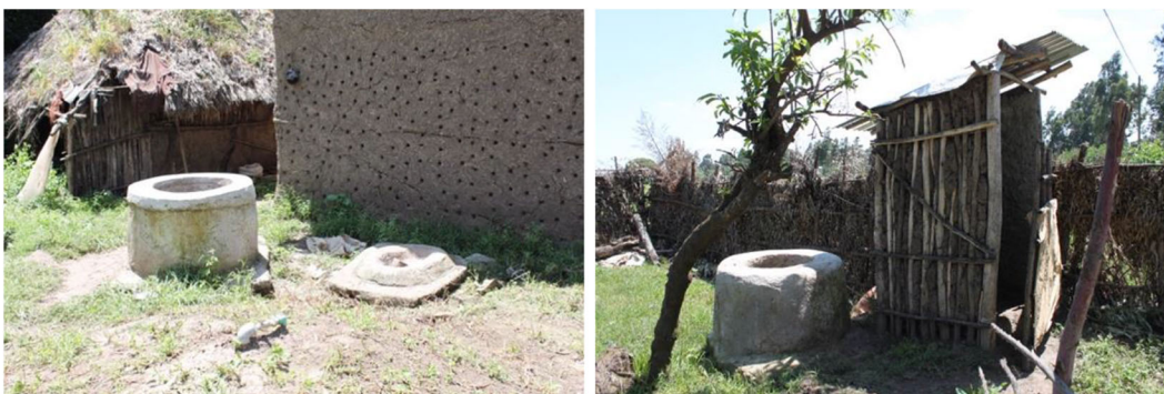
Picture 5 A latrine without a shed compared with with a shed. Source: Own
