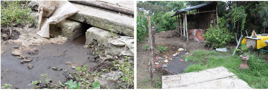
Picture 7 Poor managed bioslurry as a result of overflow and impurities. Source: Own
